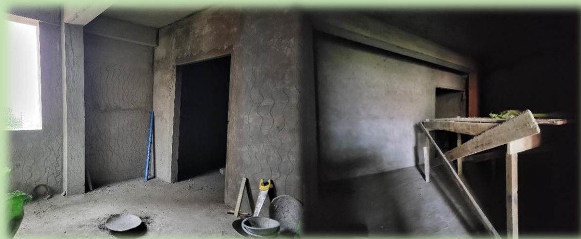
Cataract Surgical Room under construction
